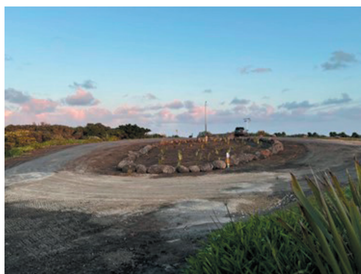
'Before and after' of the roundabout at Bourke's Lookout
